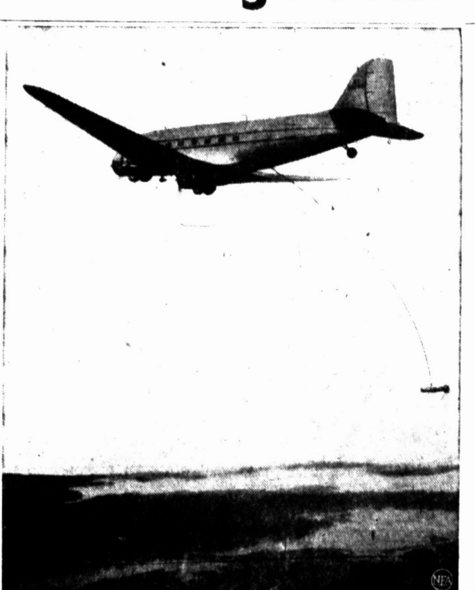
PLANE PROSPECTS FOR OIL—This airplane is prospecting for oil, using a newly developed airborne magnetometer. The instrument, which the plane trails as it demonstrates over Westchester Airport, N. Y., measures varying intensities of the earth's magnetic field. These are recorded in the plane, and data, which would take decades to gather on the ground, is quickly mapped.
