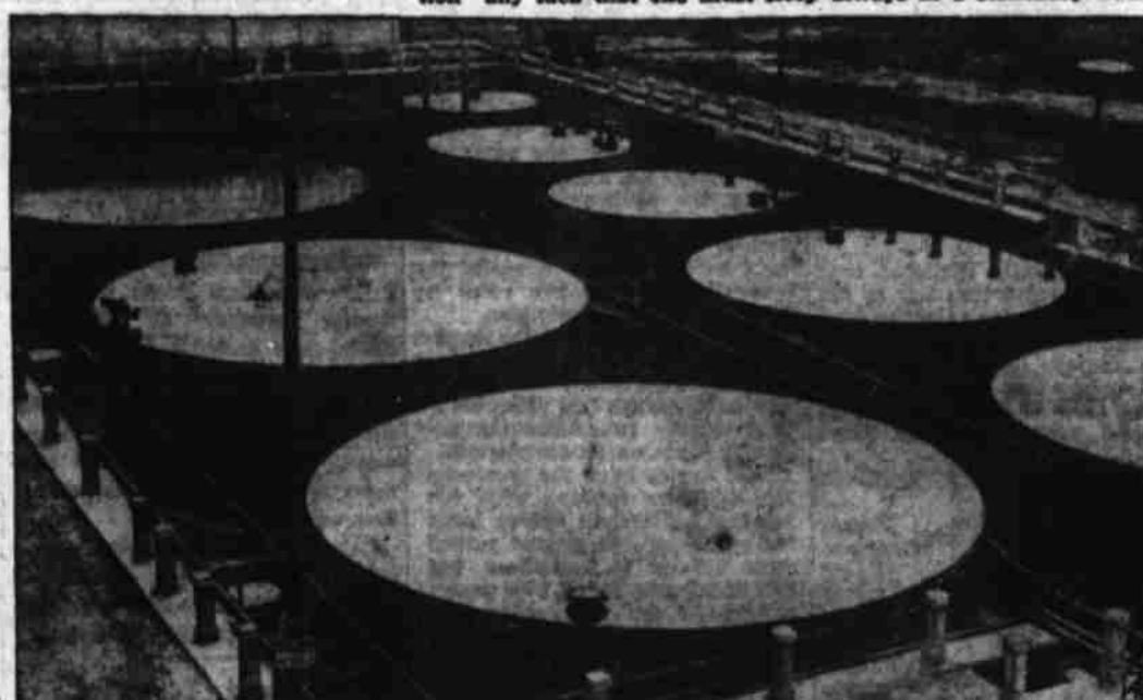
STORAGE AT BAKU. —Russia's most important oil fields are at Baku on the Caspian, where these kerosene storage tanks are pictured. Germans are believed anxious to take Baku.
