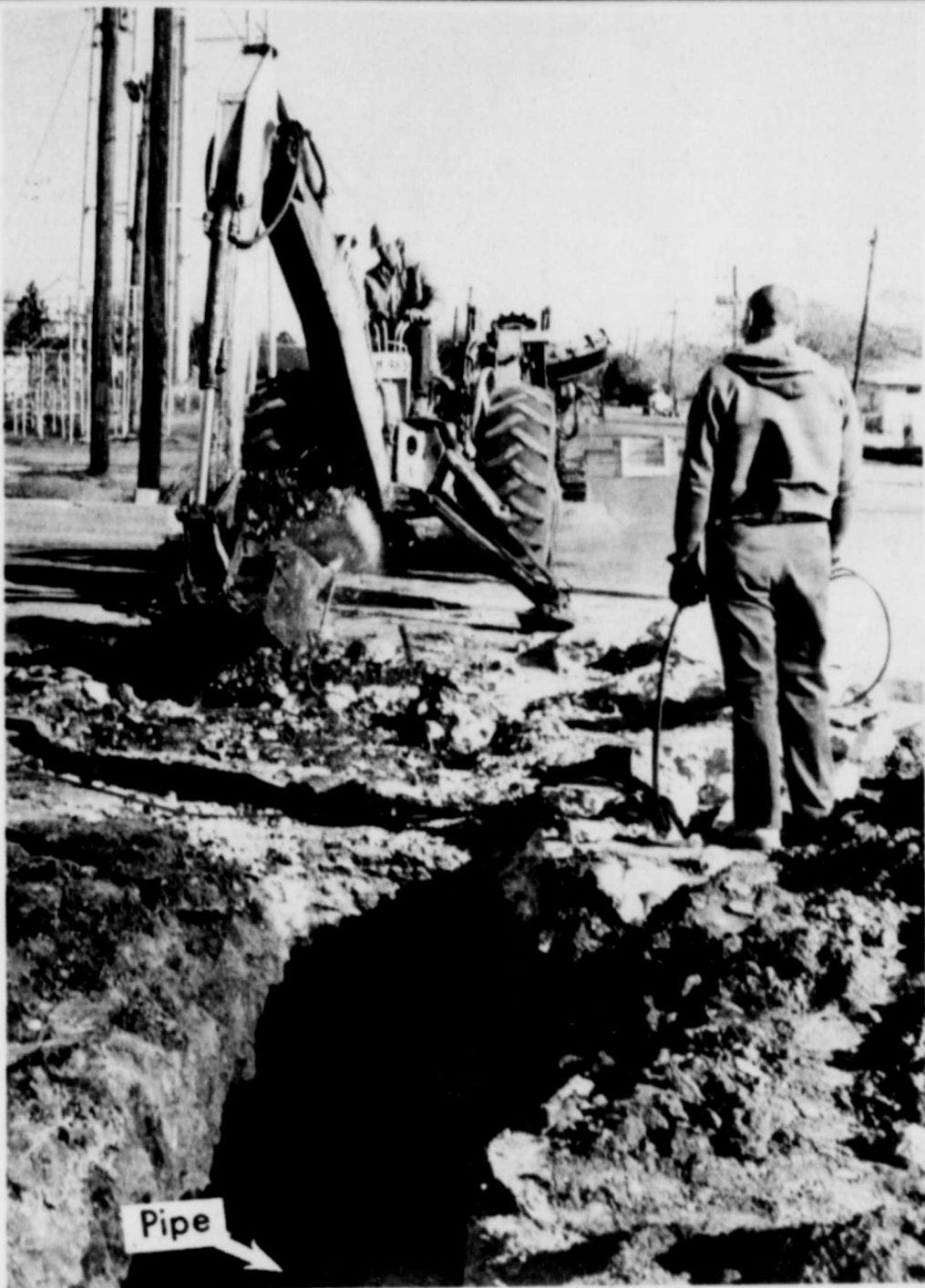
PIPELINE NEARLY COMPLETED . . . Pipeline from Wichita Falls for Burk Burnett's new water facility is nearing completion this week as several men are shown making way for the pipe on Kramer Road. The pipe portion of the facility should be completed around Dec. 15, and the water tank portion tentatively, March is the delivery date for the steel to be used on the tank. When the steel arrives it will probably take approximately twenty days to complete the project.
