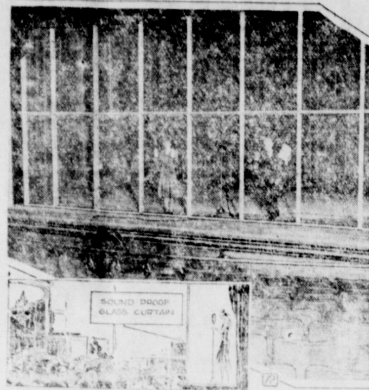
The glass-enclosed stage of the new NBC studio in New York. The "curtain," which weighs six tons, shuts off noises of the audience.
