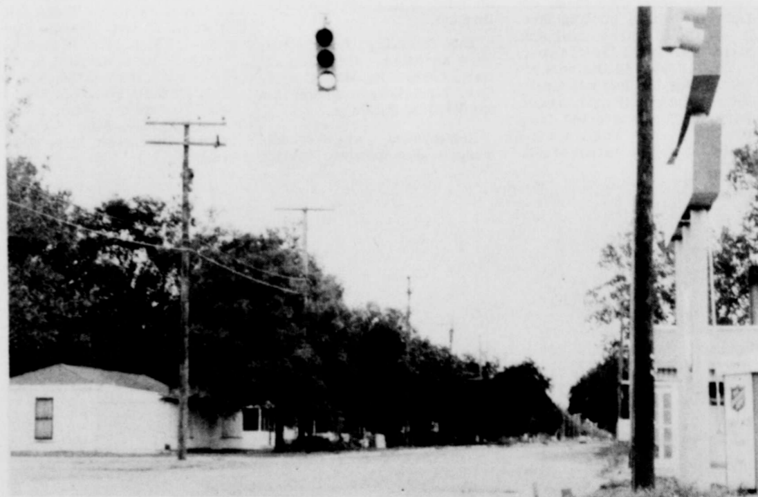
Tidal Street improvements make big difference in Burkburnett appearance.
