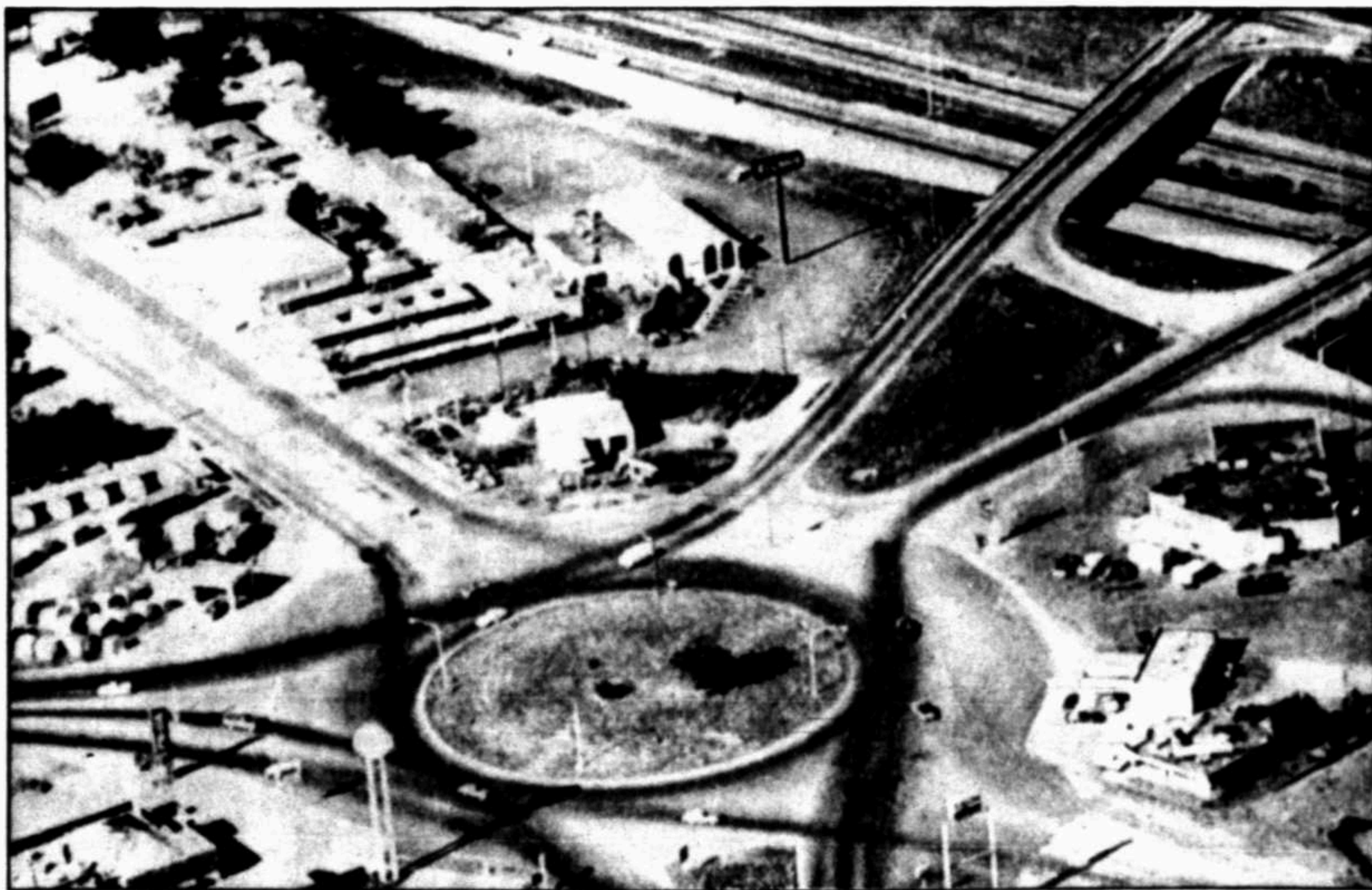
An aerial view of Waco's traffic circle, above, shows the five routes which converge at the intersection. At left, one-way signs and highway markers guide motorists around the circle.
