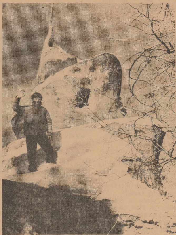
NO, IT'S NOT A TROLL'S ABODE or a gingerbread house. It's the Ensculptic VII, a polystyrene foam house that builder Stuart Gordon (above) hopes to market on a mass scale. The house costs about a third of what normal structures cost and Gordon believes that its curved surfaces will make dwellers happier.
