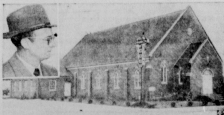
SINGLE-HANDED —Preacher John D. Smith (insert) started all by himself to build this church in East Ridge near Chattanooga.
