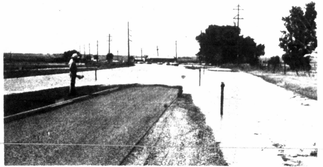
ROADS became rivers Monday afternoon for several hours after some two to three inches of rain fell within an hour's time in the Buford area. Some small hail was reported with a number of terraces broken by the runoff. Rains Monday and Tuesday supplied needed moisture for cotton planting in most areas of the county but some areas are still dry, especially in the west and southwest portions of the county.
