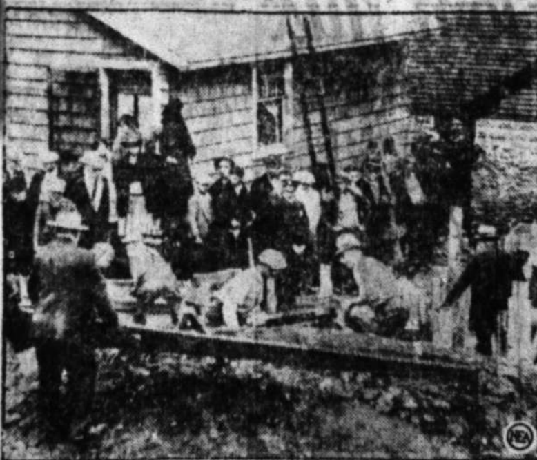
When Fred Lencow, well-digger, was trapped by a cave-in forty feet down a well at Westport, Mass., police and firemen sank a parallel tunnel and saved him after 29 hours' imprisonment. You see the feverish work in progress here.
