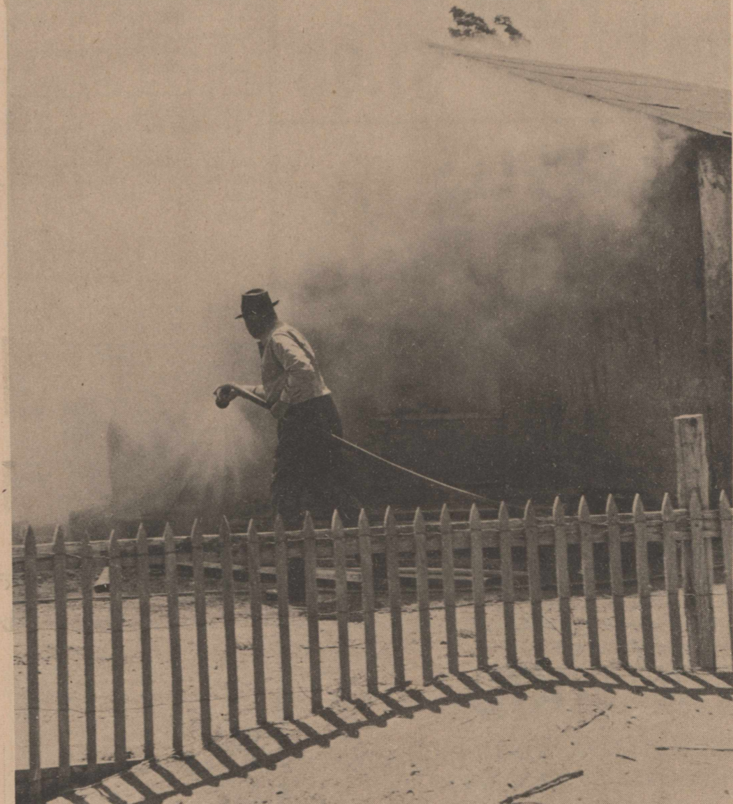
THIS TWO-room structure and home of Jose Garcia and family was "guttered" by fire Tuesday about 11 a.m. Firemen were called after flames were already visible through the roof. The house was declared a "total loss". The fire was believed caused by faulty electrical wiring.
