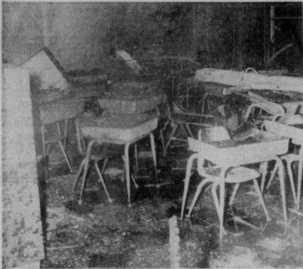
CLASSROOM RUBBLE —Desks and other equipment were left in ruins following an early-morning fire at Stanfield Elementary School. Damage to the building and equipment has not been calculated.
