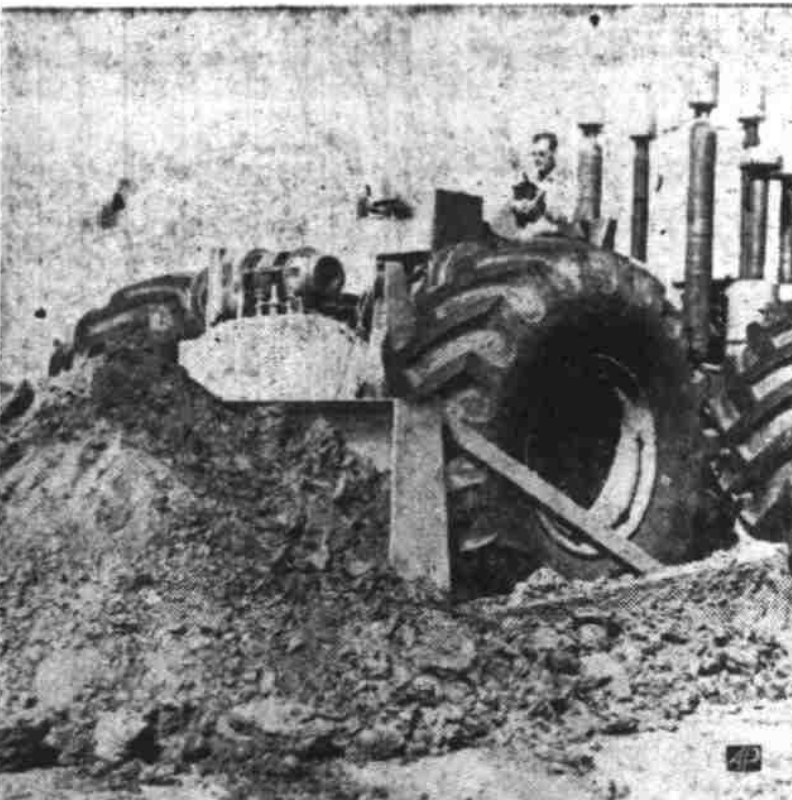
BIG BULLDOZER — This huge bulldozer, a 90,000-pound giant, is shown at the plant of the manufacturer in Longview. The machine was shown for the first time at the Greater East Texas Industrial Exposition in Kilgore. It rides on 93-inch high rubber tires and is called "The Pipe Organ" by the men who built it. (AP Photo).
