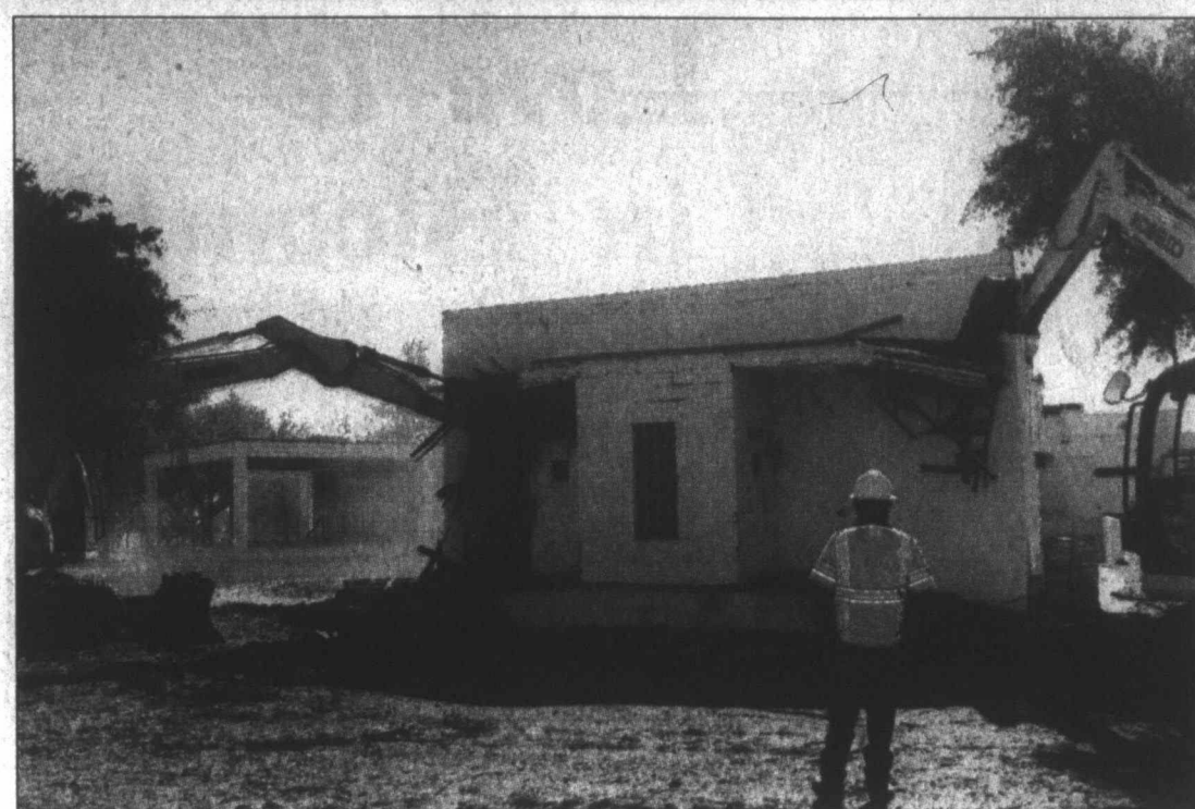
TEARING IT DOWN —With Bill Ellis looking on, the first demolition of the old hospital building on Chestnut Street began last week with a crowd watching. MCHD Administrator Robbie Dewberry held a ceremony to give citizens a chance to say goodbye to the structure that housed the hospital for over 70 years.
