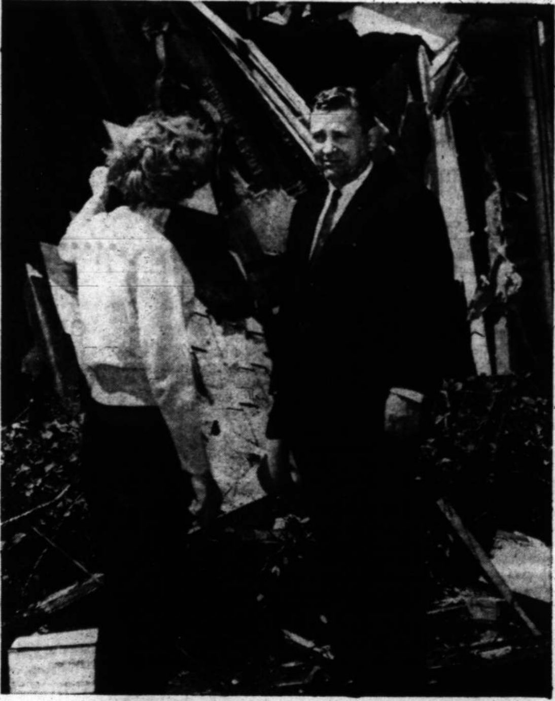
VIEWS STORM DAMAGE — Texas' senior U. S. Senator Ralph Yarborough discusses condition of one of the Lincoln Heights houses severely damaged in Friday's twister, with a resident of the area. Shown is portion of a railroad boxcar which was blown through the front of the brick house. Yarborough was in Wichita Falls for three hours Sunday viewing the damage. He left for Washington at 1:25 p.m. after pledging his assistance "in any way I can" to help erase the ravages of the storm. (Staff Photo)
