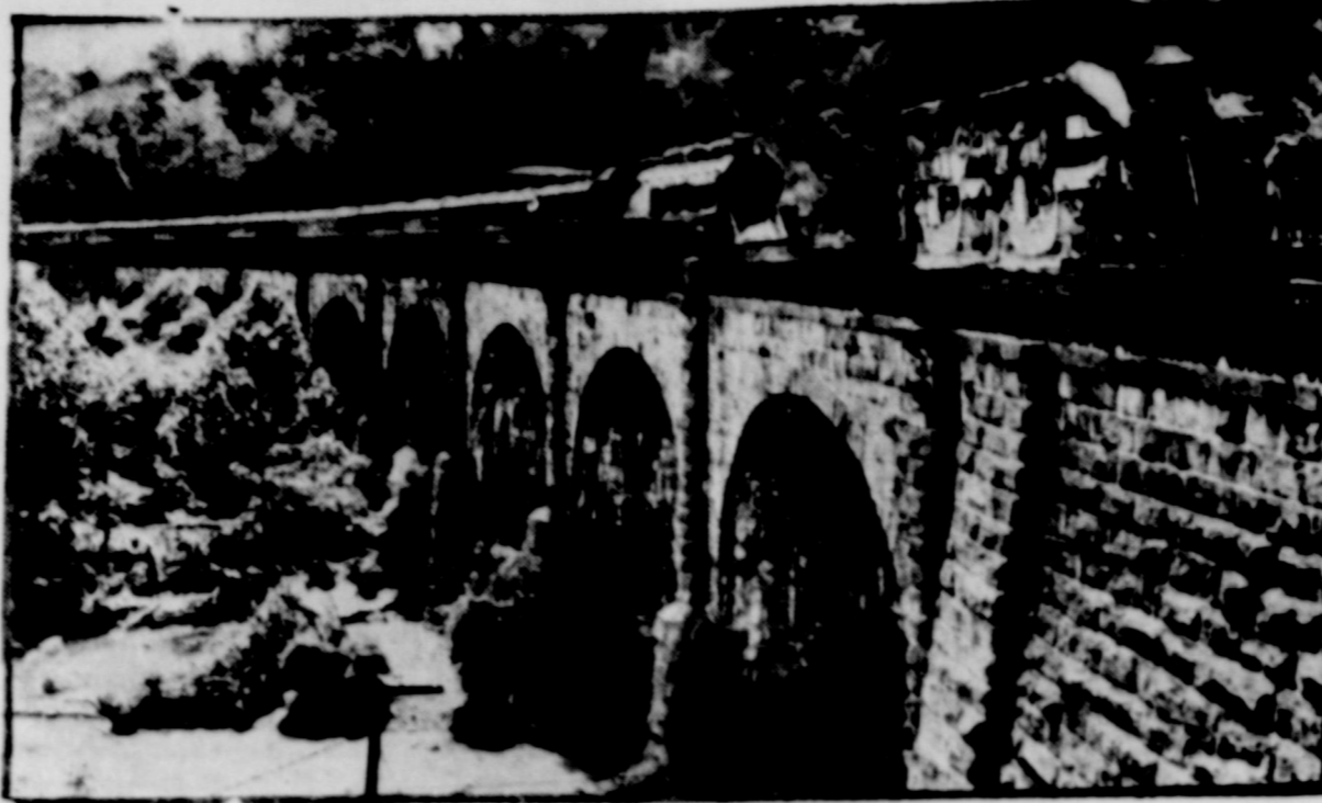
At Relay, Md., stand a viaduct that has rendered 100 years of steady daily service carrying the heaviest trains. It is the Thomas viaduct of the Baltimore & Ohio line, the oldest of its kind in the world, spanning the Patapsco river outside of Baltimore. The 103-year-old Atlantic locomotive and Inlay coaches in use in the 1830s are here contrasted with the streamlined train—the Royal Blue—that began using the bridge the other day on the Washington to New York run.
