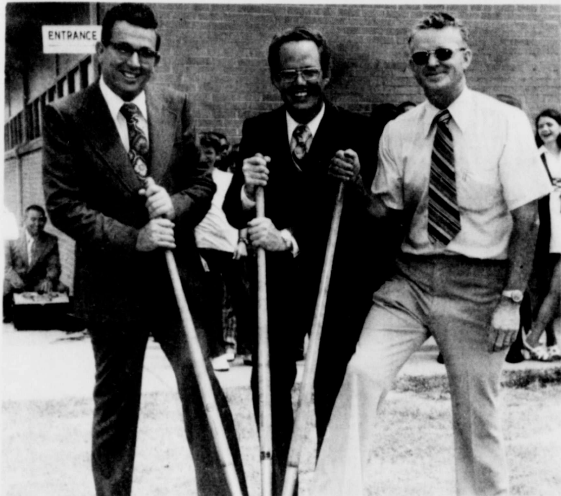
An official ground breaking ceremony was held last Sunday morning at 11:30 a.m. at the Central Baptist Church, directly following worship services. The ceremony marked the official beginning of construction on Central Baptist's new $122,000 educational building. Shoveling the first dirt are (left to right) Joe Ray McCluskey, building contractor; Max Dowling, pastor of the church, and Cotton Kinnard, chairman of the building committee. Central Baptist Church is located at 814 Tidal Street in Burkburnett.
