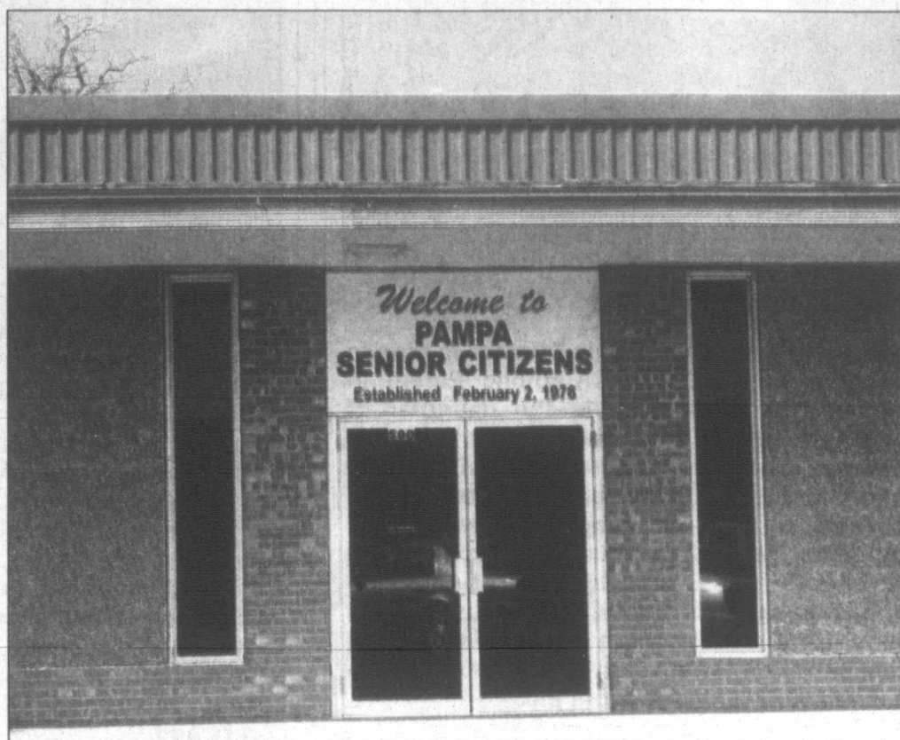
Pampa Senior Citizens Center opened Feb. 2, 1976, at 500 W. Francis, the site of a grocery store which was bought and renovated to use as a center.
