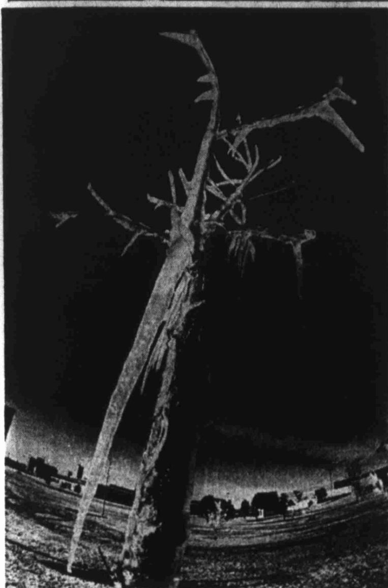
SANTALAND FROZEN — A malfunctioning sprinkler system created an icy wonderland Wednesday morning in what had been Santaland at the eastern edge of the civic center complex. A spokesman for the city parks and recreation department said no permanent damage to shrubbery resulted. (Staff Photo by Jim Watkins)
