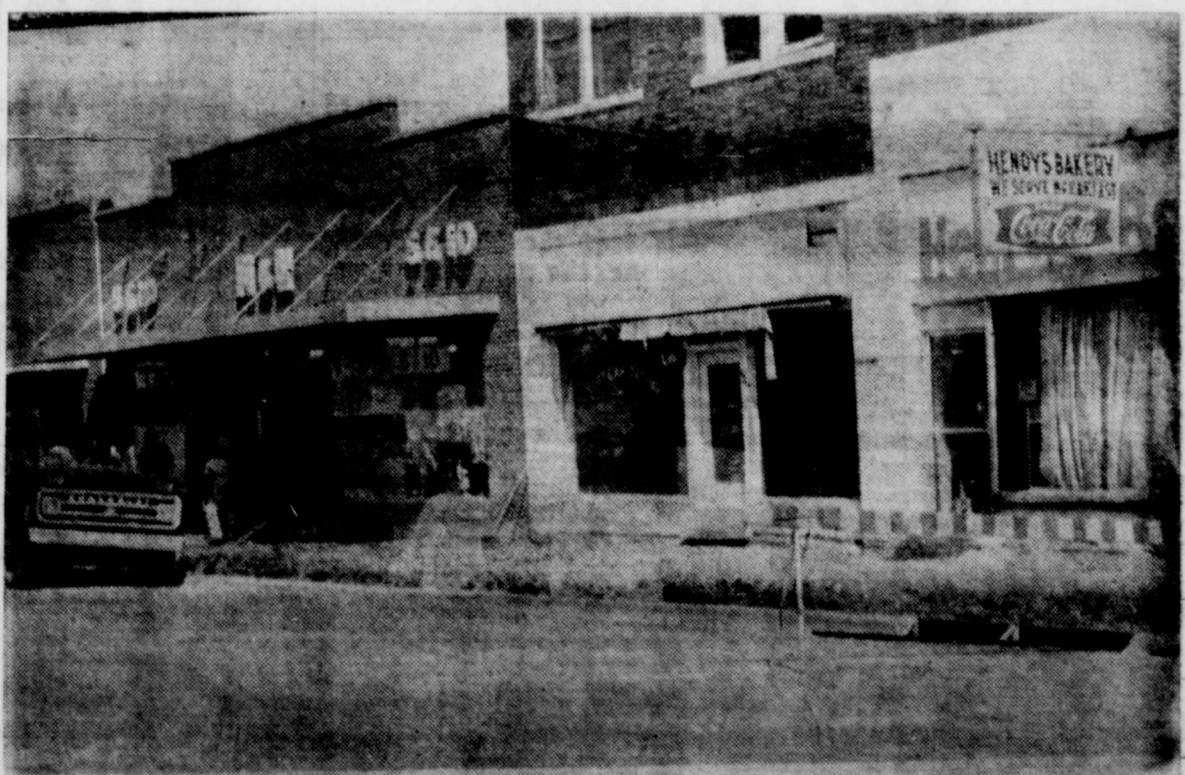
NEW SIDEWALKS AND GUTTERS have been installed on a section of Third Street by city crews. Sidewalks, from Henry's Bakery to M&N 5&10, were
