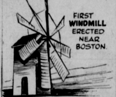
FIRST WINDMILL ERECTED NEAR BOSTON.
