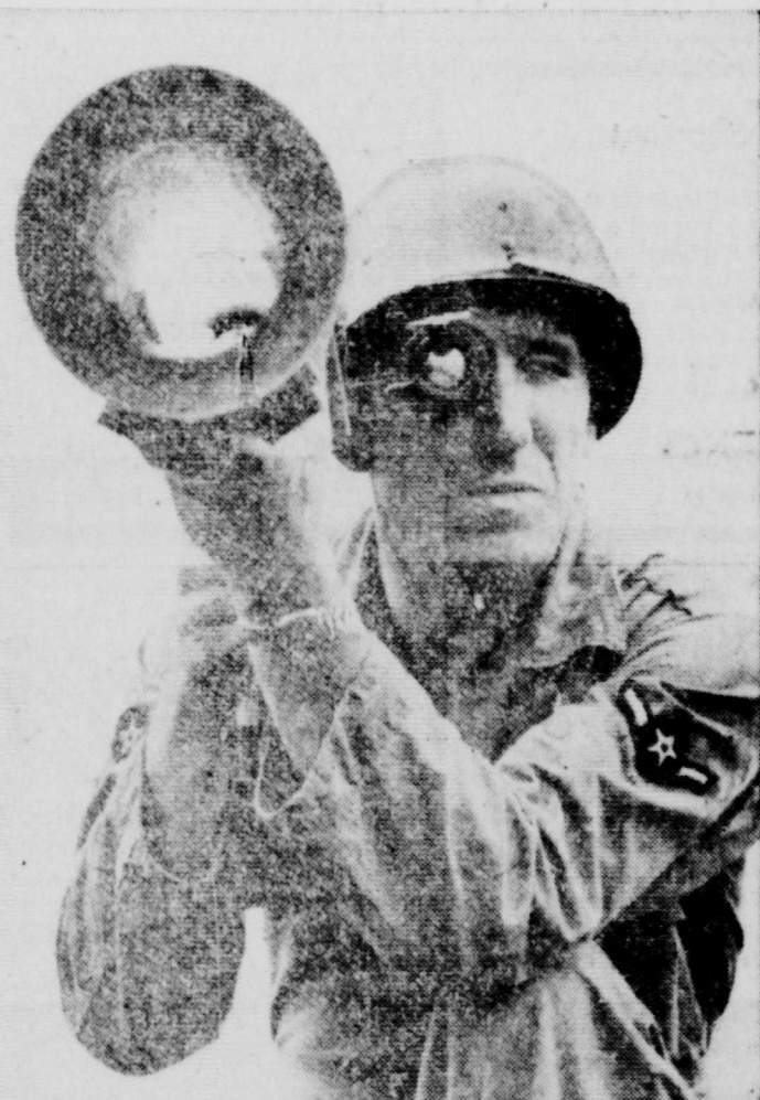
SUPER BAZOOKA —The 3.5-inch rocket launcher now being used in Korea is held by Matthew J. Keppinger in Aberdeen, Md. Be- lieved to be one of the most effective anti-tank weapons because of its ability to penetrate 11 inches of armor plate, the launcher is five feet long and weighs 15 pounds. It fires a nine-pound rocket by means of a small electric magneto in the trigger mechanism.
