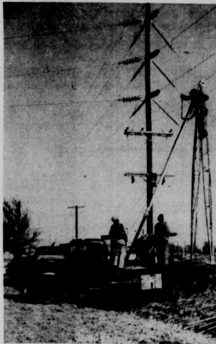
NEW LINE FOR BUILDING—Community Public Service workers are shown getting a new line ready to serve the Texas Highway Department warehouse on highway 117 just west of Perryton. The earth work is being done now for the new building, and when the structure is completed, the highway department will move from their site south of town near the city lake. Shown above, on the derrick is Mike Jackson, while like Kennedy and Short Symons are on the truck.
