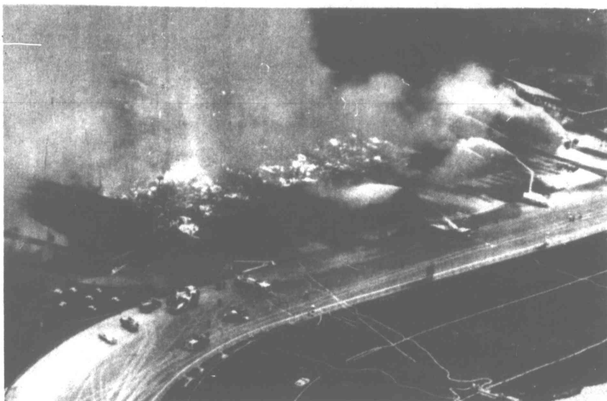
FIERY SCENE — Fire trucks work from the race track, foreground at Garden State Park in Cherry Hill, N.J., Thursday as the grandstand is leveled by flames. More than ten thousand persons were in attendance when the blaze started.
