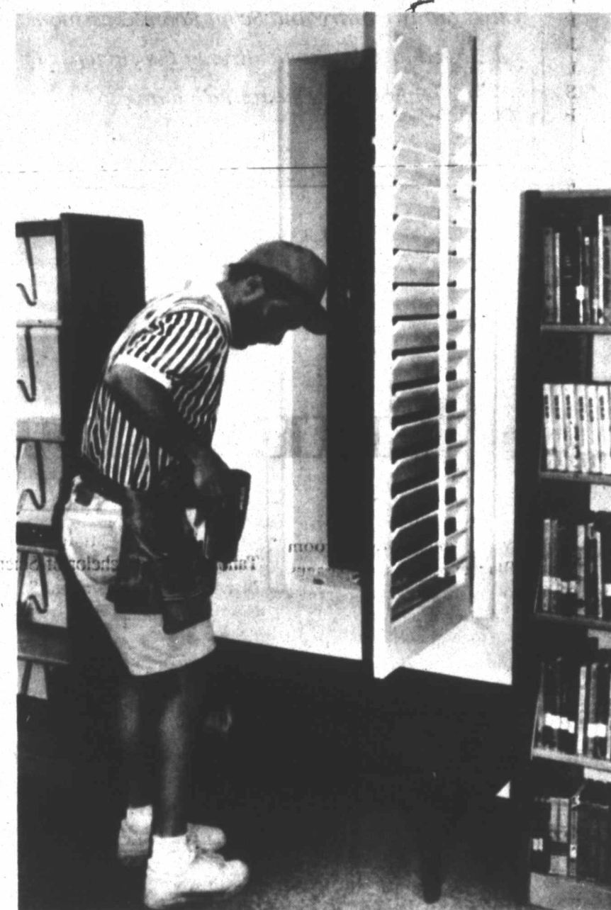
HANGING SHUTTERS - Ken Brown of Tahoka works on hanging one of the new shutters at the Life Enrichment Center, which he completed last week. This window is in the new library. Brown, a craftsman who works for a shutter company in Lubbock, made the plantation shutters by hand, sanded and finished them and installed them on all the windows in the new center, all as a voluntary donation for the Life Enrichment Center. (LCN PHOTO)
