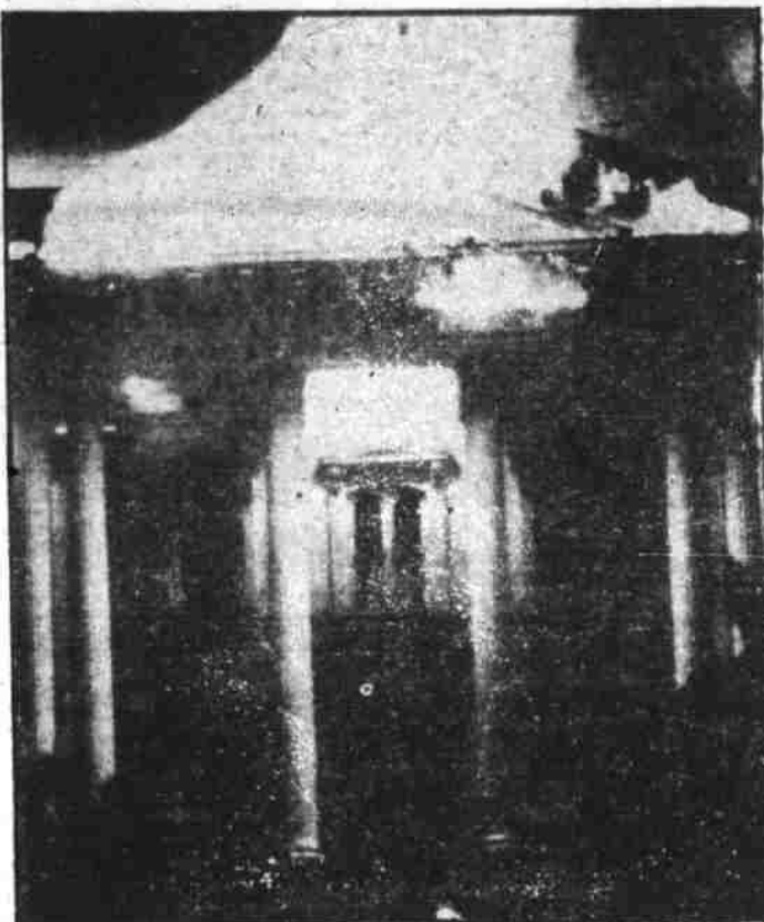
This night photograph shows the blazing Oregon state capitol at Salem, shortly before the dome of the 60-year-old structure collapsed. One fireman lost his life in the blaze, estimated to have cost $2,500,000. (Associated Press Photo)
