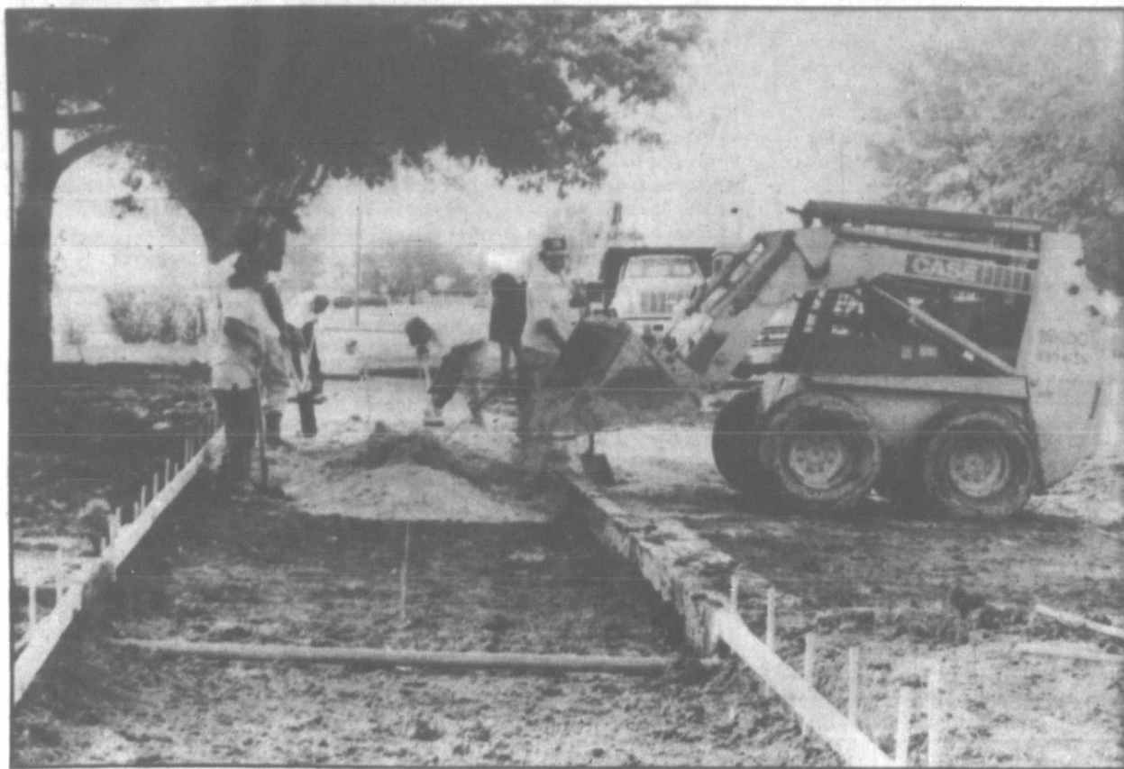
Workers prepare the base for a new sidewalk going in place on the west side of St. Matthew's Episcopal Church this week. In addition to replacing the sidewalk, the church also is having a new water sprinkling system installed for its lawns. The sidewalk is being constructed by Hargrove Construction, and Jack Curtis Well Service is installing the sprinkling system. (Pampa News photo by Darlene Holmes)
