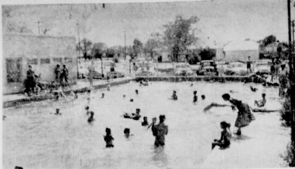
HOT DAYS are swimming days for many Lockney youngsters and some older people as well. Here is a scene from the Lockney swimming pool
