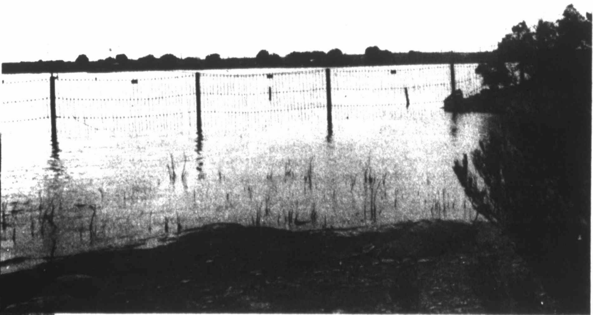
The lake side area of the discharge area is guarded by a strong cable fence to keep boats out of the area.
