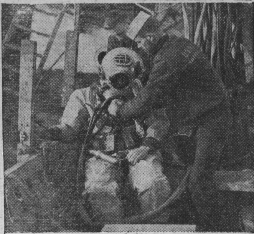
The U. S. Navy is now clearing up the Bay of Naples for Allied shipping. The Nazis attempted to block every berth by sinking ships and barges and toppling cranes and even nearby buildings into the water. This photo shows a Navy diver, F. F. Garrigues, of Camden, N. J., being undressed by two other Navy men after a dive into the bay. (Official OWI photo—Rural Press Section)
