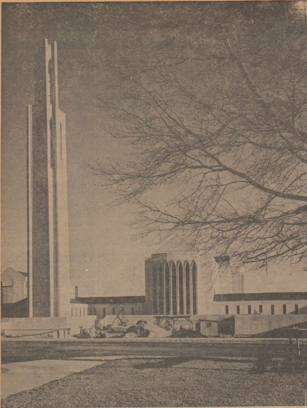
THE NATIONAL PRESBYTERIAN CHURCH AND CENTER, now 85 per cent completed, is expected to be finished by this summer. The complex covers about an acre in floor space in Washington, D. C. A 173-foot tower dominates.
