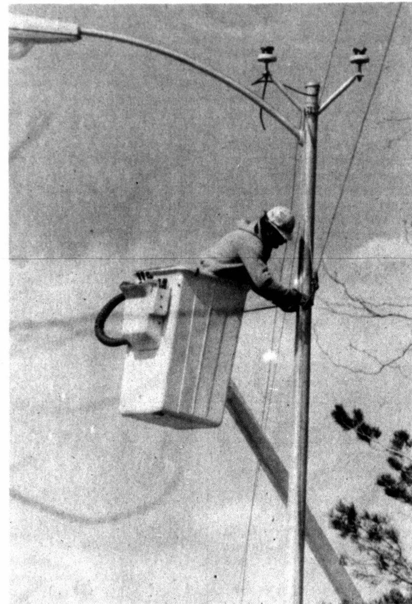
Randy Heckman with Southwestern Public Service Co. works on stringing new line Monday in the 900 block of North Hobart.
