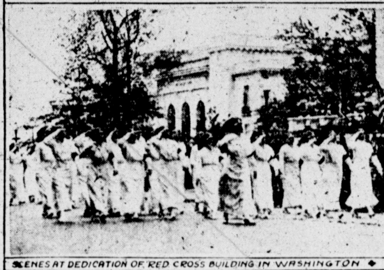
SCENES AT DEDICATION OF RED CROSS BUILDING IN WASHINGTON
