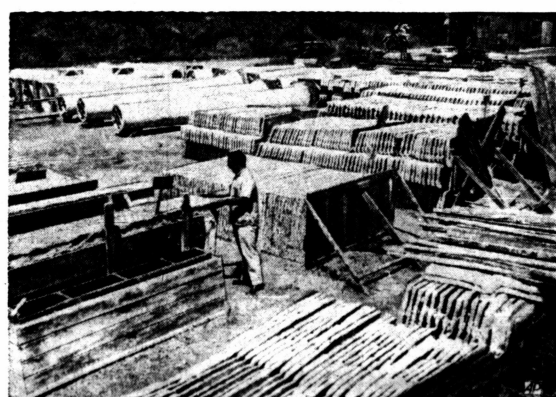
MOVIE MAGICIAN AT WORK — Plaster craftsman Rudy del Pardo checks over sections of plaster "stone" which will be fitted into pattern of walls, houses and shopfronts on biblical movie set being constructed in Hollywood, Calif.
