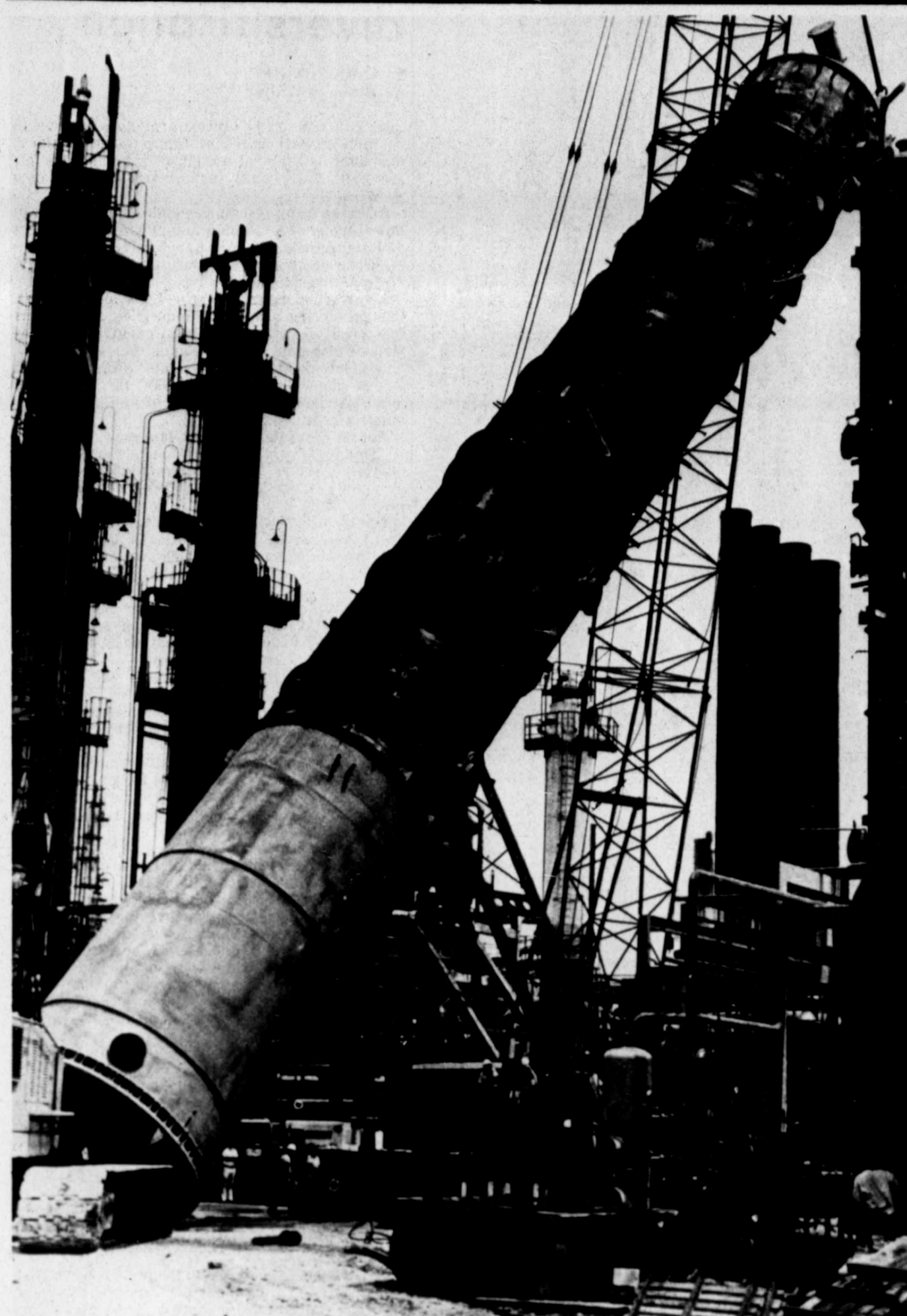
This gas oil fractionator is representative of the enormous pieces of equipment required at Amoco Texas Refining Co.'s oil refinery in Texas City. Weighing 180,000 pounds and measuring 130 feet
