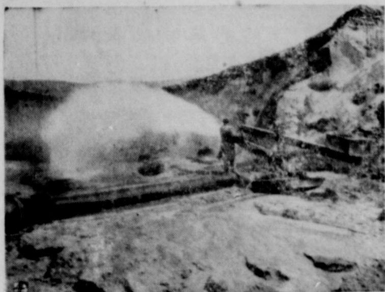
BEACH MAKER —Giant nozzles spray sea water on dunes near Los Angeles beach, washing sand into the ocean. The city of Los Angeles is building a new beach, extending the present footage from 100 to 600 feet in order to take care of more California bathers.
