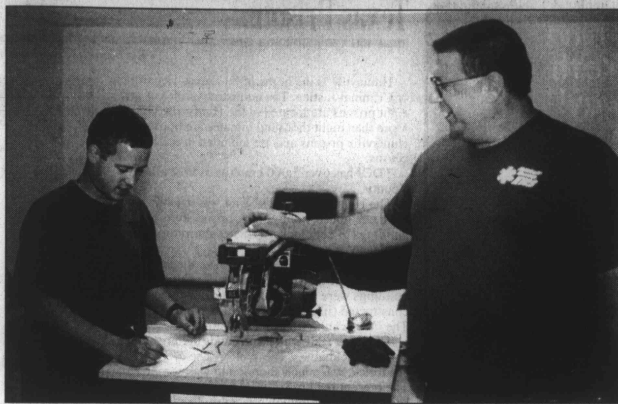
MITCHELL COUNTY EMS Director Mark Potter, right, talks with one of his paramedics, Shane Terry, during work to renovate their new East Hwy. 80 office building.
