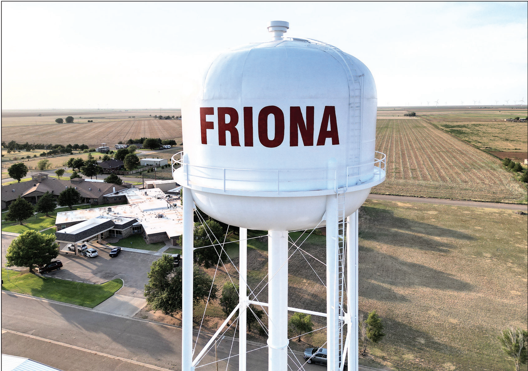
Friona’s refurbished water tower is soon to be back online. (Photo for Friona Star by Randy Geries)
