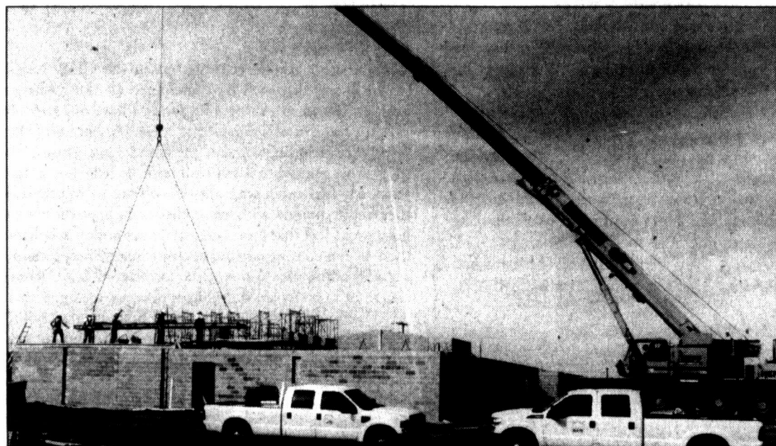
Mickey Neff, CFO of Neff Crane and Rigging, LLC, was on hand Monday at the site of Mitchell County's new law enforcement center. Josh Brady was operating the big 100,000-ton crane placing cement ceiling panels on top of a portion of the new jail. Neff said he had three cranes larger than the monster working at the jail. Neff said they would be unloading a total of 25 trucks of the panels this week, with nine trucks on two days, including Monday, and seven on another day.
