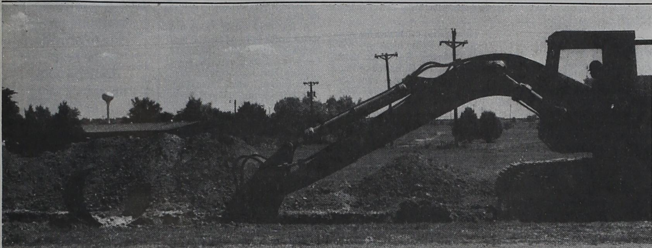
DIGGING AWAY —The construction of the drainage system on NW 11th and NW12th Streets began last week. Traffic was temporarily blocked on these streets as well as the Country Club entrance while the pipe was being laid. These drainage pipes will discharge 1,000
