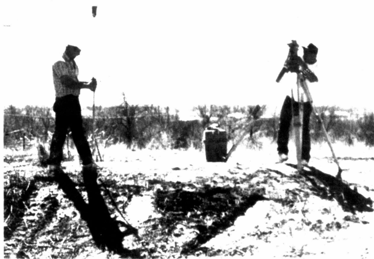
SURVEYING — Wilson Surveying Company of Lubbock has had a team in Snyder to begin preparations for a topographical map of the existing wastewater plant. The map will then be used
