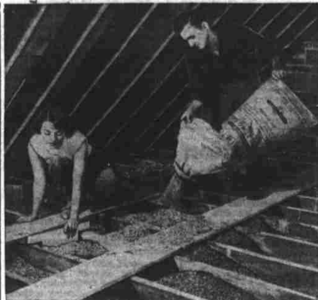
MODERN INSULATION is lightweight. Here a Chicago couple pour vermiculite between attic joists to demonstrate how easy it is to do the job yourself.
