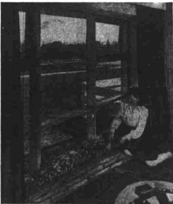
THE CALIFORNIA-STYLE window, formed by a 2 by 4 framing, which is strong enough to support double sealed insulating glass, is now popular even in the smallest homes. This is a design by Rudolph A. Matern, architect.
