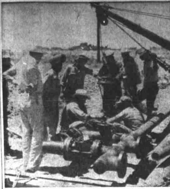
Making The Tie-In
