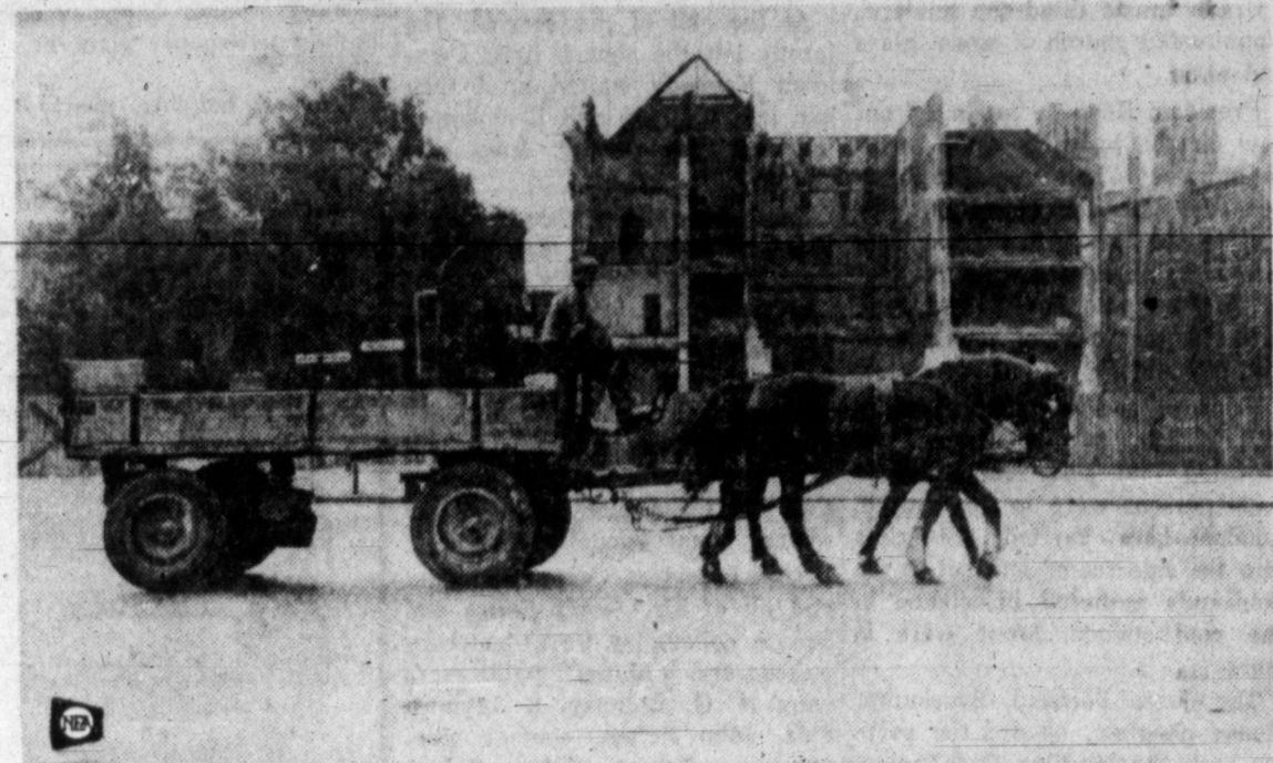
TIRED, DREARY EAST BERLIN — Rebuilding a church near Stahloff Platz (right) cannot obscure the ruins that have been in disrepair since World War II.
