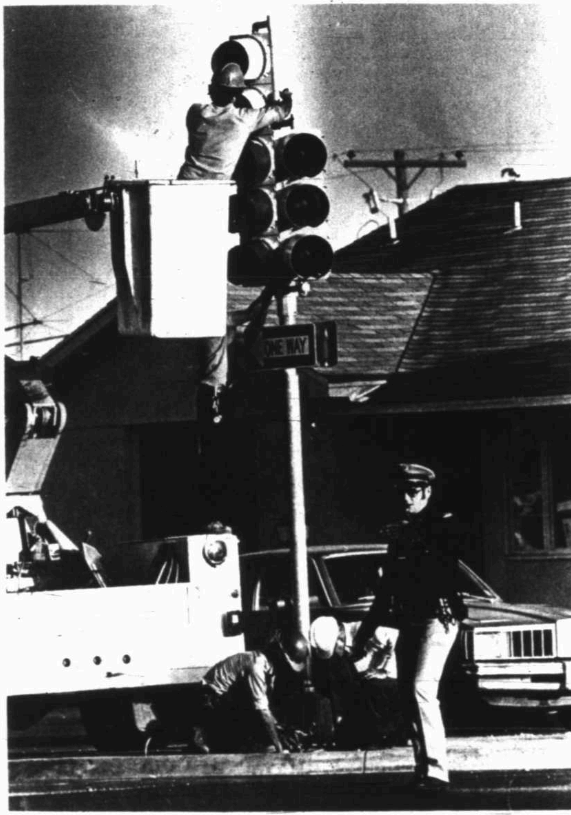
A city policeman directs traffic Monday while city employees finish installing a traffic light at the intersection of Michigan and Louisiana. The light was necessary for moving traffic on the portion of Michigan from Louisiana to Andrews Highway that has been changed to one-way traffic going east.
