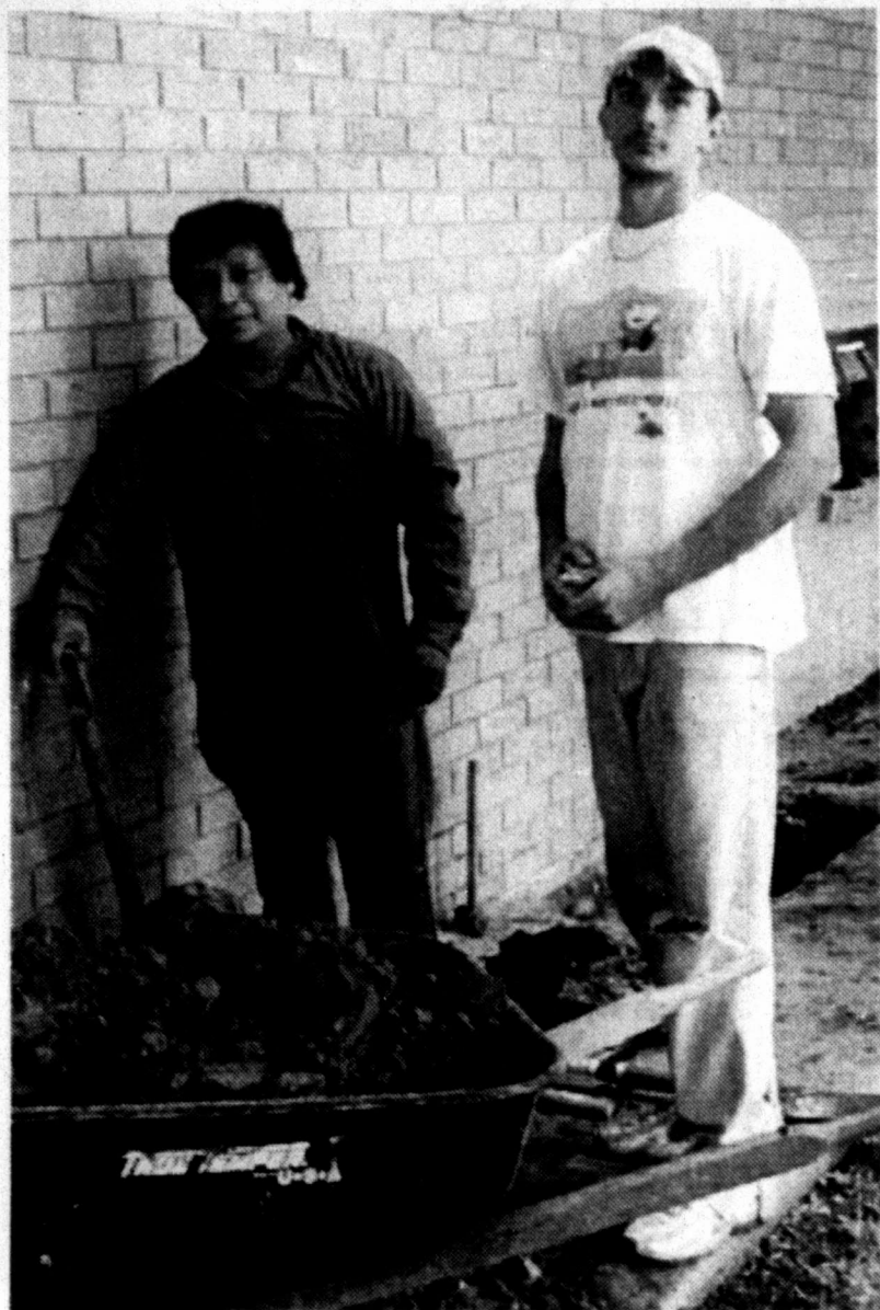
LIBRARY PROJECT CREWMEN Hermillo Martinez Olmos of Vera Cruz, Mexico, and Cody Nevels of Abilene show some of the 36 inch holes they will fill with concrete to stabilize the building.
