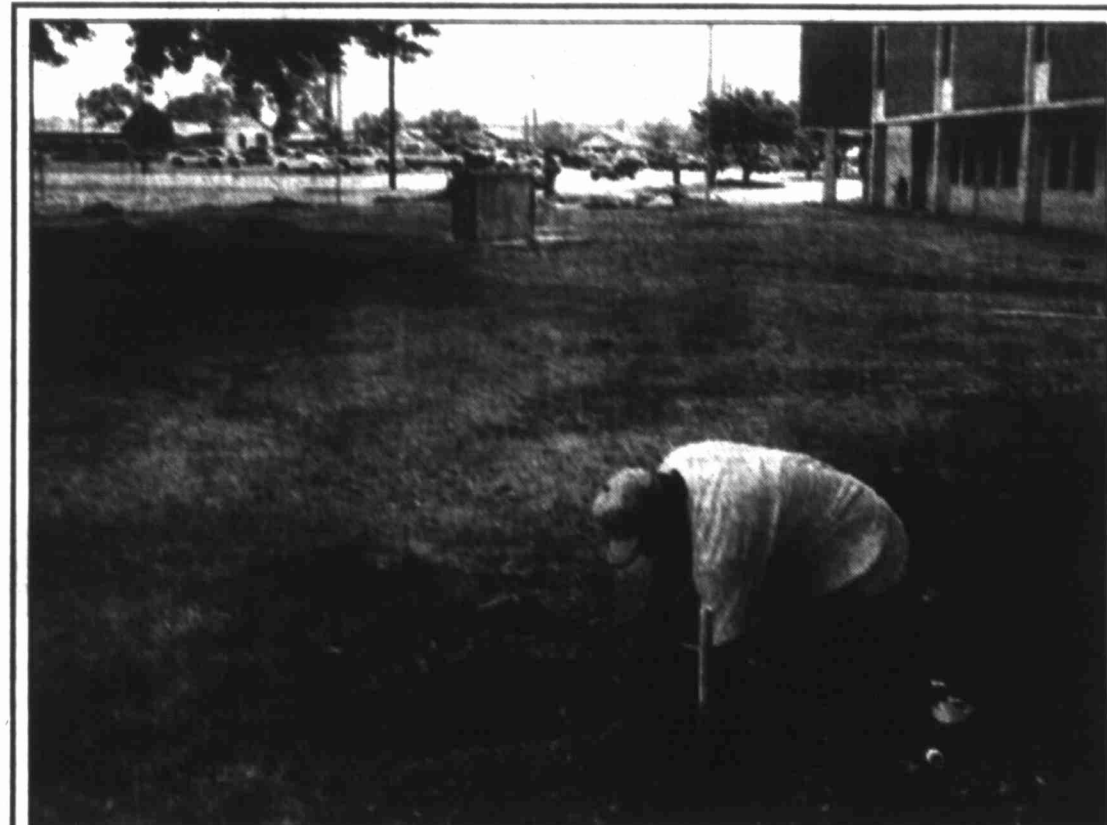
Big Spring ISD maintenance worker Able Cruz works on part of a sprinkler system that is being installed at the high school. The mulberry trees lining the front of the school are being uprooted in order to place the sprinkler system in the ground.
