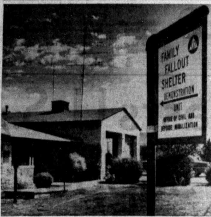
The Sign Locates The Shelter
