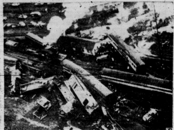
OHIO TRAIN WRECK—This aerial view shows the wreckage of a New York Central passenger train which left the rails at Wellington, Ohio killing four persons and injuring scores more. The smoke is coming from the wrecker clearing the tracks. (AP Wirephoto.)
