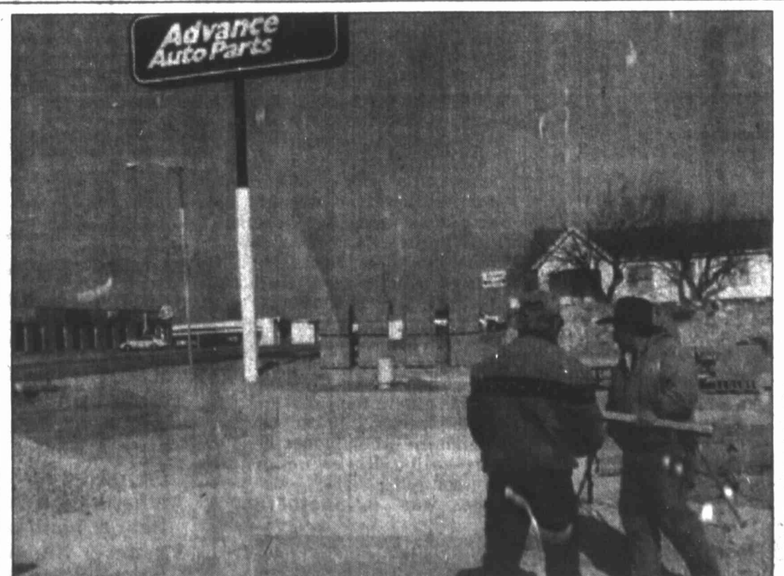
HERALD photo/Andreas Modlin Ground work continues at the site of the Advanced Auto Parts store, located at the corner of Gregg and Seventh Street. Construction has been delayed due to weather but the steel framework is expected to be up by Monday.
