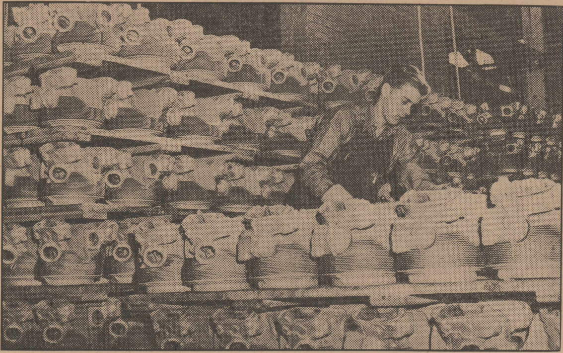
Row on row of rapidly produced airplane cylinder heads stand as symbols of speed-up in American defense production. They are being made at Wright aircraft plant in Fairlawn, N. J., America's first-line production foundry devoted exclusively to molding and casting of cylinder heads.
